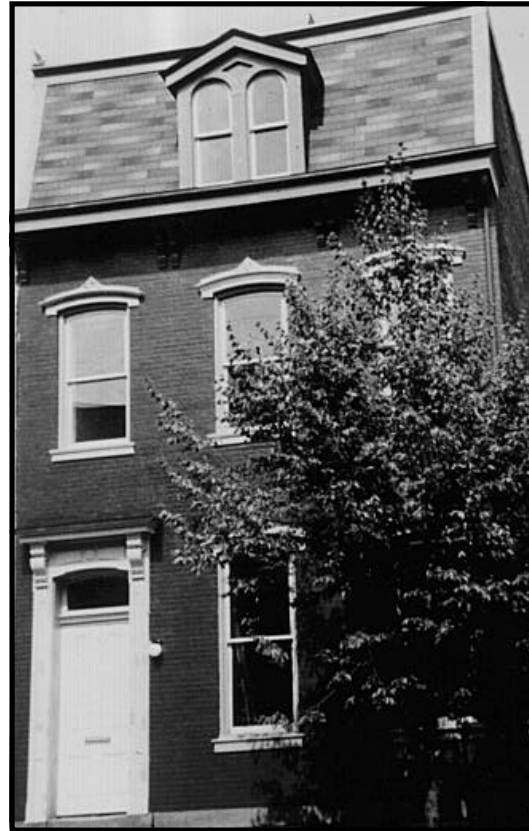
Figure 18.2 Historic Property After Lead-Based Paint Was Chemically Removed.
