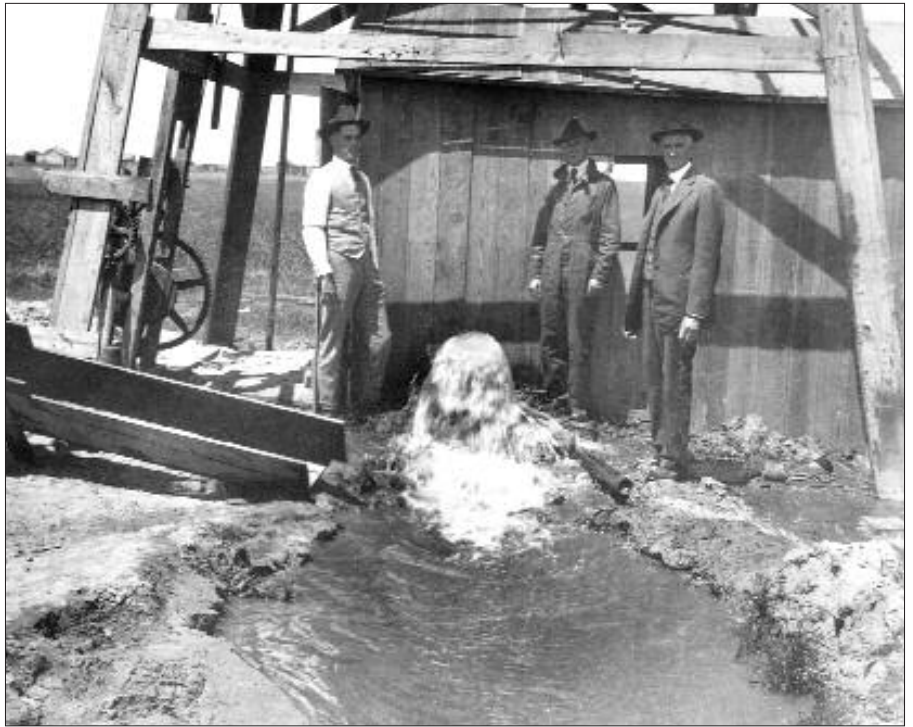
Men at a pump house and irrigation ditch in Seward County.
