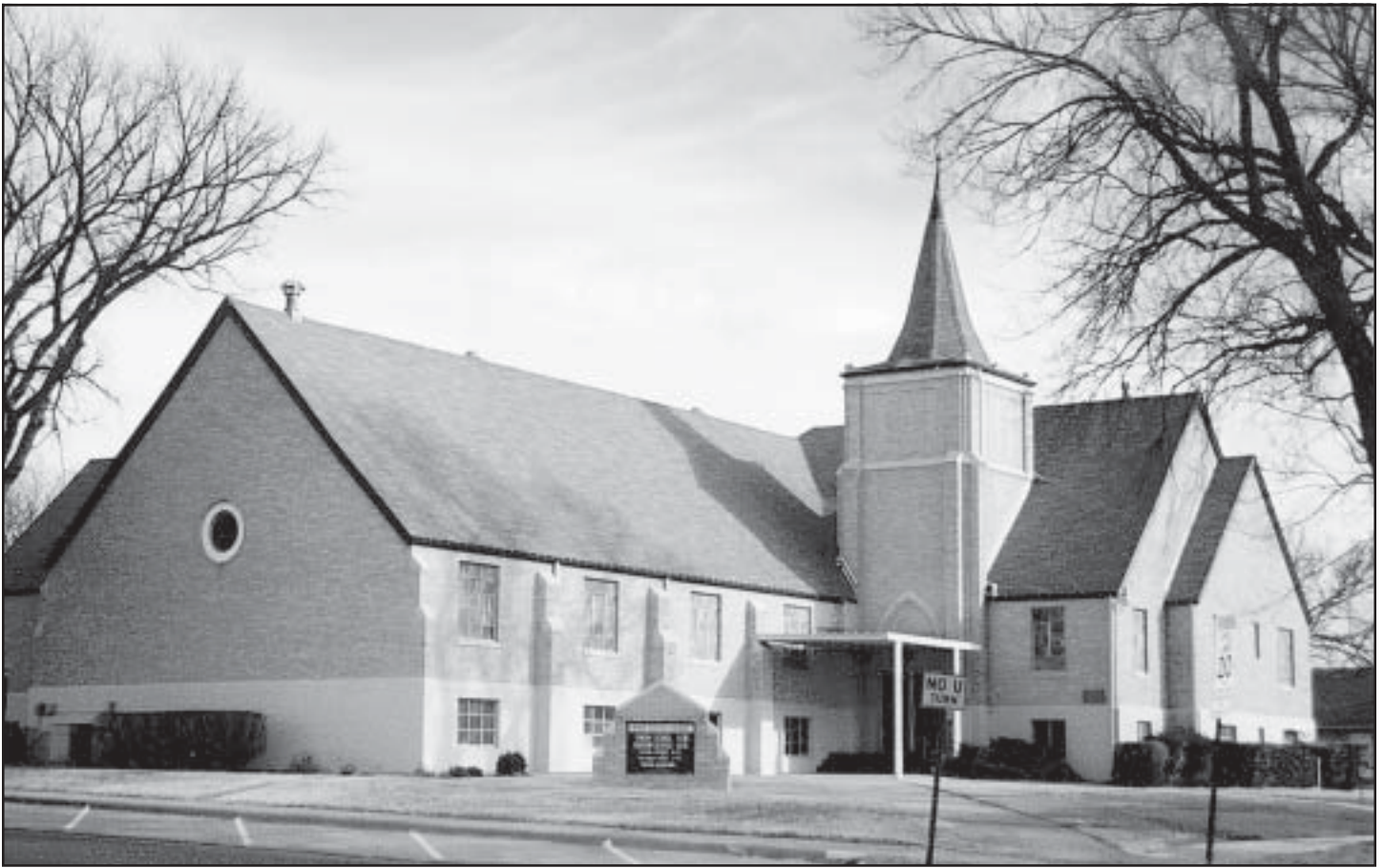
First Baptist Church in Kingman, which was dedicated in 1953, is a vernacular structure that combines mock buttresses and a Gothic arch over the entrance with the square nine-pane windows common to buildings in the middle of the twentieth century. The light brick was another common feature of mid-century construction.
