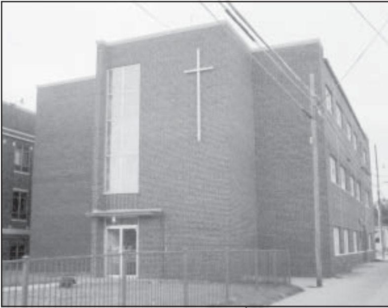
(Left) While the main sanctuary of First Christian in Wellington is in a classical design from the early twentieth century, its education wing has the simple lines, plate glass, and metal window frames from the 1950s.
