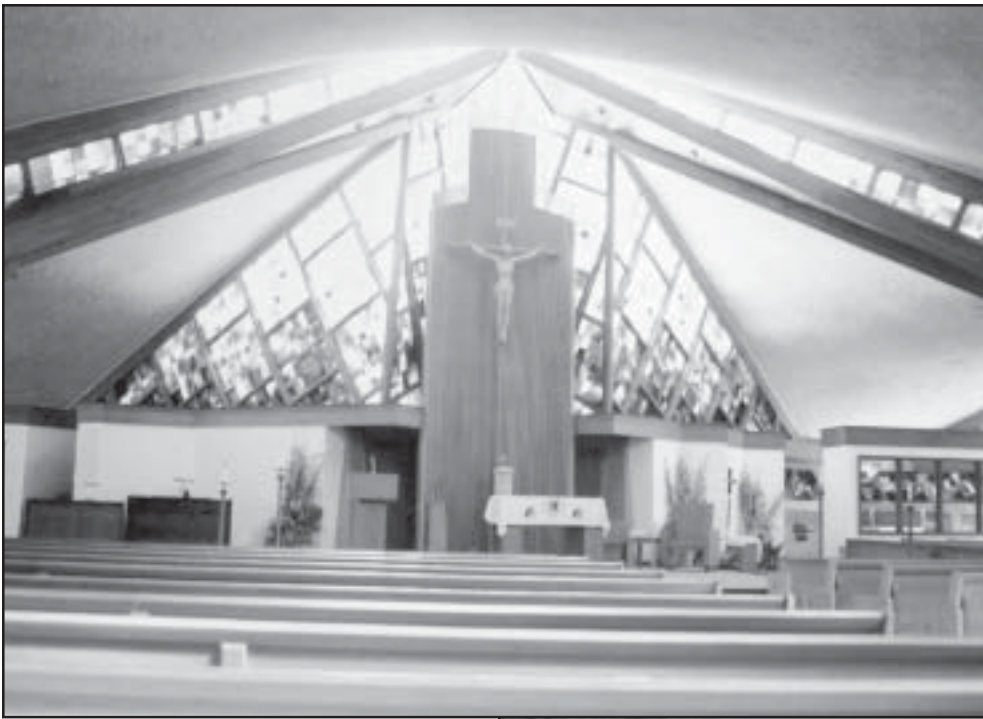
The design of the Mary, Queen of Peace Catholic Church in Ulysses used hyperbolic paraboloids for the roof, concrete for the walls, and stained glass for the spaces in between. The floor plan is more of an auditorium than a traditional basilican arrangement.
