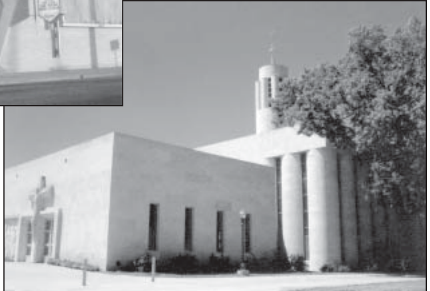
(Right) Edward Schulte designed Salina's Sacred Heart Cathedral to reflect the look of grain elevators. The walls for both the inside and the outside feature the concrete of which they are made.
